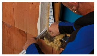
**5. Install the window and insulate the joint** Fold in the CONTEGA SOLIDO SL and install the window properly. Use a suitable fastening system. Fill in the joint with a suitable approved insulation material, leaving no cavities.
