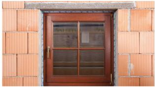
**4g. You're finished!** The airtight joint is now complete, and the tape can be plastered over.
