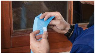
**1a. Remove the inner release film** Remove one of the release film strips on the membrane side (smooth side).
