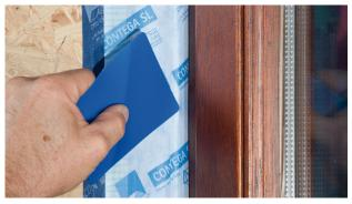
1e. Rub the tape firmly to secure the adhesive bond
