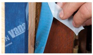
**1d. Stick to the reveal** Remove the second strip of release film from the smooth membrane side and stick the tape all around the reveal.
